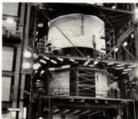
Upper portion of the Saturn "stack" being readied in the VAB.
